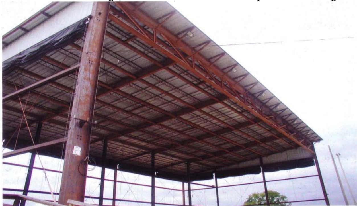
View of the roof structure and hanging grid for lighting and sound.
